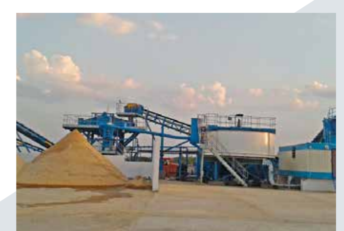
Stage Two – On site processing
